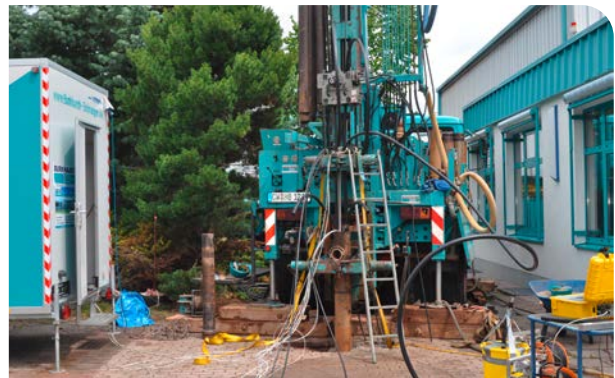
The image shows a geothermal probe drilling with integrated measuring technology on the company premise of Burkhardt GmbH.
