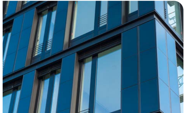
The ZSW has mounted a test facade to their new institute building in Stuttgart to gather operating data of the modules.
