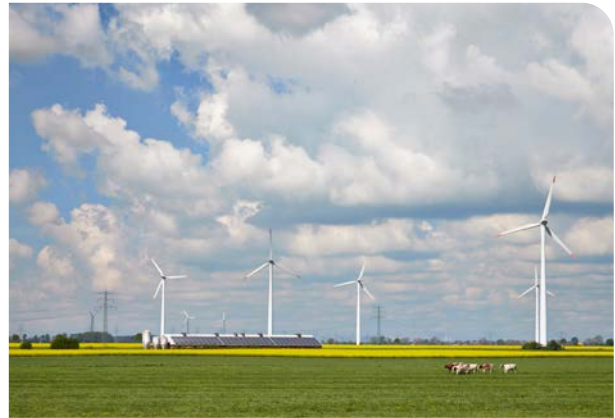
ENSURE develops reliable power grids for the sustainable energy supply of tomorrow.
