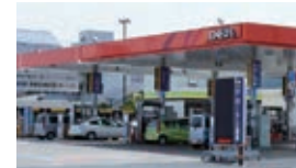
2012 Commercial model demonstration hydrogen station constructed
