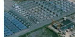
1986 Experiments on a large-scale grid-connected photovoltaic power system started for the first time on Rokko Island in Hyogo Prefecture
