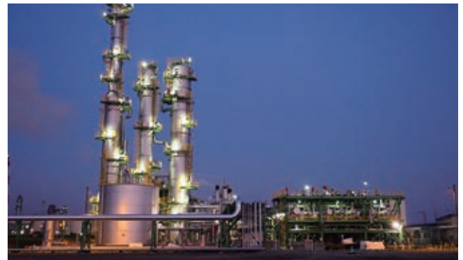
Tomakomai CCS Demonstration Facilities
